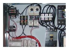
The programmable controller allows for customized programs to better meet customer needs. The controller eliminates the need for relays and timers that take up valuable panel space. All electrical components are UL and CUL listed.
